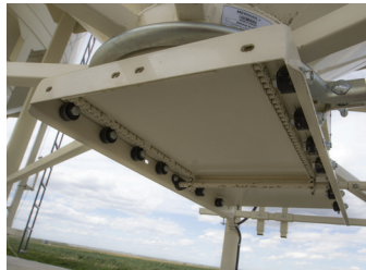
Rack-n-Pinion slide gate
